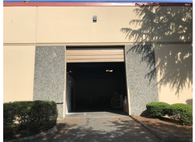
One grade level loading door (14') on side of Building
