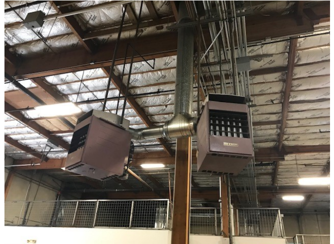
3 Gas Heating Units in Warehouse
